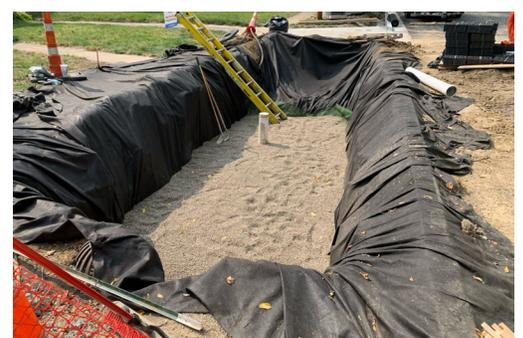
Steve Krehbiel, Quick Supply and our engineer, Bill Murphy, assisted with the installation of a FocalPoint high-performance modular biofiltration system for this project.
