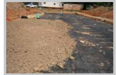
Fig. 20 Pushing backfill parallel to the Geogrid prevents the grid from shoving.
