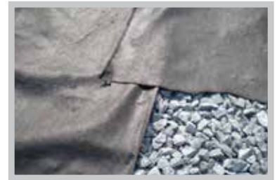
Fig.4 Reduced overlaps don't create significant savings and can create delays.
