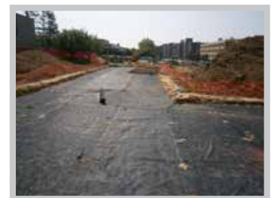
Fig. 19 Overlap Geogrid 18" or as required by plans.
