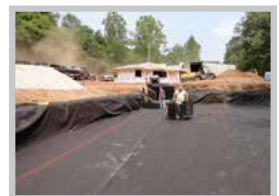
Fig. 5 Use a string line and marking paint to square the system footprint.
