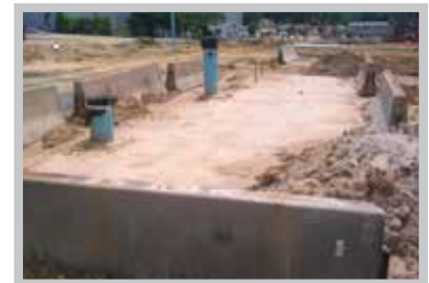
Fig. 22 Secured R-Tank® installation using Jersey Barriers.
