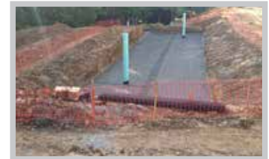
Fig. 21 Secure the installation with temporary fencing.
