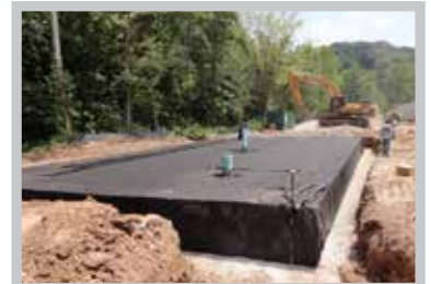
Fig. 15 Finished envelope should lay flat against R-Tank®.
