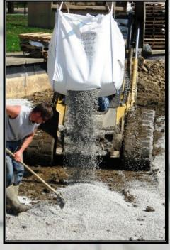
Provided the product is kept dry, AquaBlok® can be handled much like crushed stone aggregate. Conventional methods and equipment can be utilized to apply the material in a broad range of environments and circumstances.
