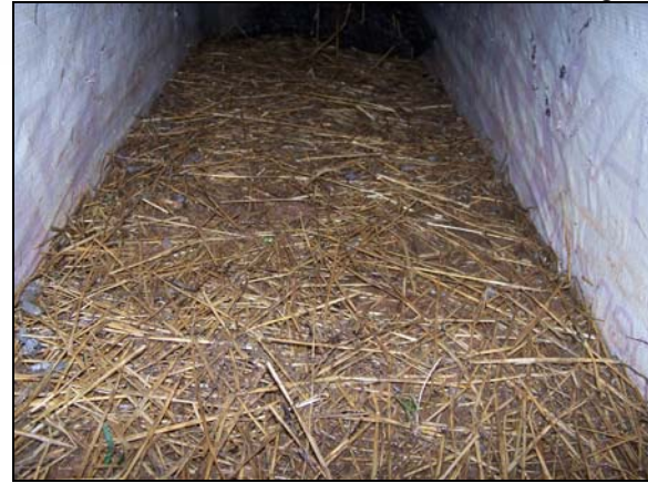
Figure 8. Channel After Matting Removed (no apparent soil surface disruption)
