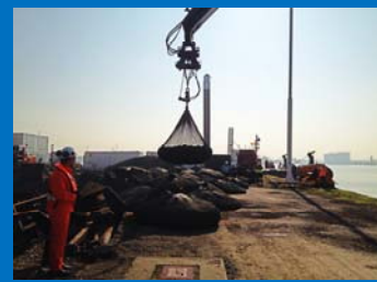
Belgium 2014 scour protection
