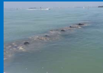
Italy 2009 create canal dike
