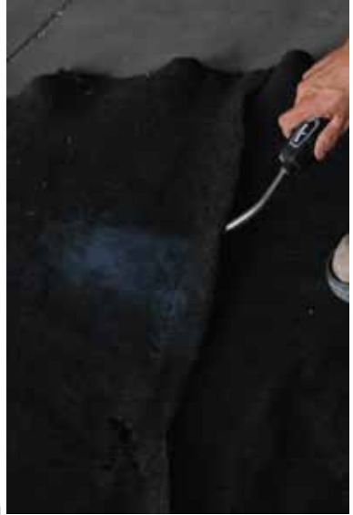
Figure 29: Geotextile being melted together with a torch.
