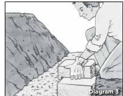
Construction of the next course
