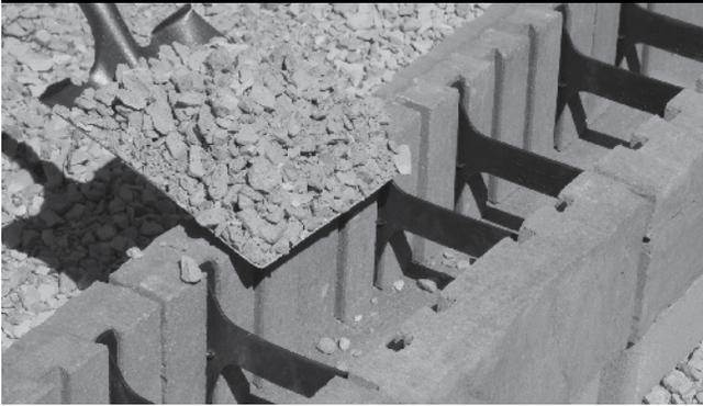
Place 3/4" crushed rock in between the panels to provide frictional connection and proper internal drainage.
