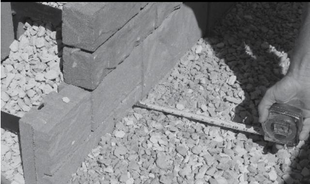
Place 12" of 3/4" drainage rock behind the rear panel of the wall. This will provide for proper drainage behind retaining walls.
