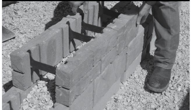
Set additional courses of the Tandem Wall. Making sure that you are keeping the wall in proper alignment. Backfill and compact each additional course.
