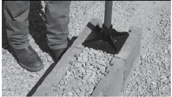
Lightly hand compact the gravel in between the panels for proper compaction.
