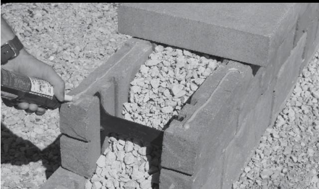
When placing the cap on top of Tandem Wall, use a construction adhesive to secure the cap to the top of the wall.
