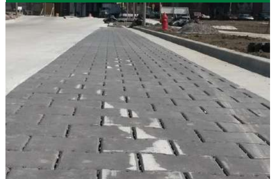
Can Plow and Seal To Prevent Salt Damage
