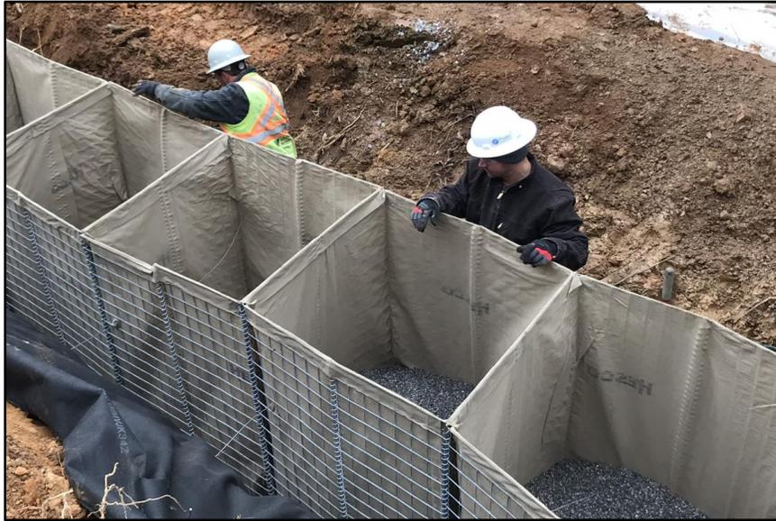
8. Install remaining fill in lifts no more than 2 ft (0.6 m). Fill the units and backfill behind the units simultaneously so as to balance the earth pressures. When normal water levels are present, face units should be filled with granular, self-consolidating material. Compact infill and backfill to the specified modified Proctor dry density per the Engineer's recommendation, but never less than 87% of the maximum dry density per ASTM 1557.
