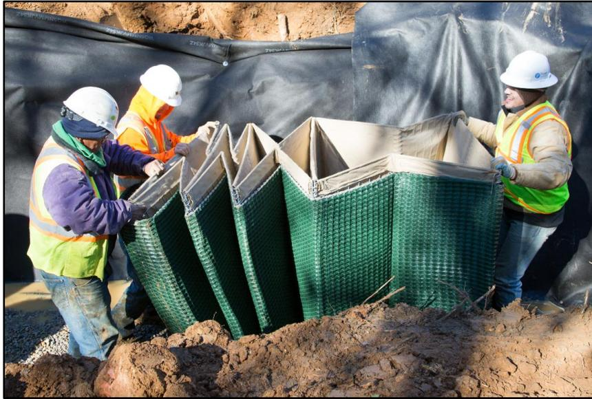
3. Gradual curves can be created due to the system flexibility. Curving is done during setup and all curved units must be set out and joined before filling. Each of the 15 ft (4.6 m) long units can be curved a maximum of 12 in (30 cm) from the tangent line set by the previous unit. Tighter concave or convex curves can be achieved as shown below.
