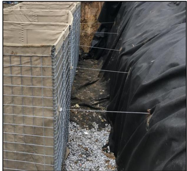
7. Place a 6 in (15 cm) thick fill material approved by the Engineer within the units. Check and adjust the units to ensure a level placement. If joining the units together in series, do not fill the end cell more than 6 in (15 cm) prior to joining units.
