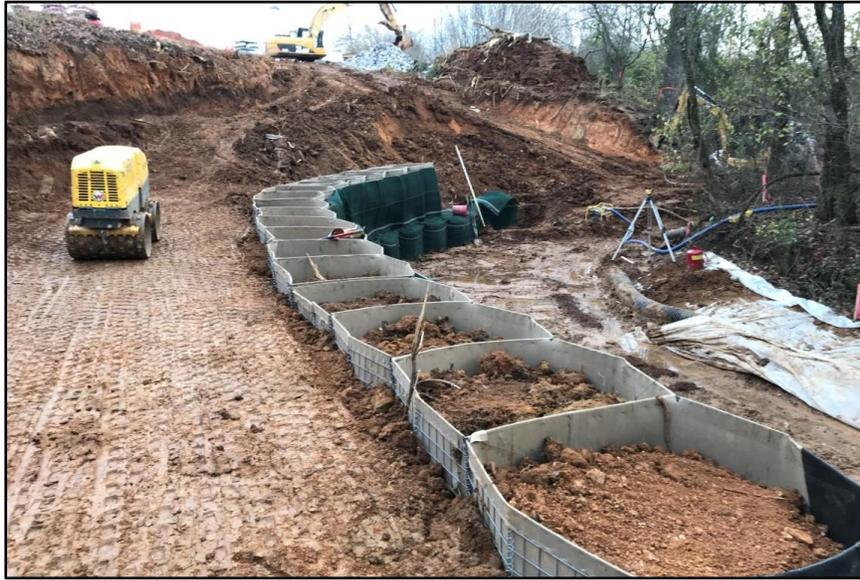
9. For vegetation establishment on the face of the units, fill the pocket between the HPTRM and the cell with seed and growth media. This can consist of 50% topsoil, 50% hardwood mulch, and seed. Place a minimum of 1 in (2 cm) of topsoil/mulch/seed mix on the top of the filled unit.
